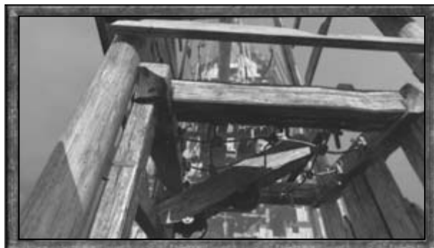
A crude yet ingenious elevator
